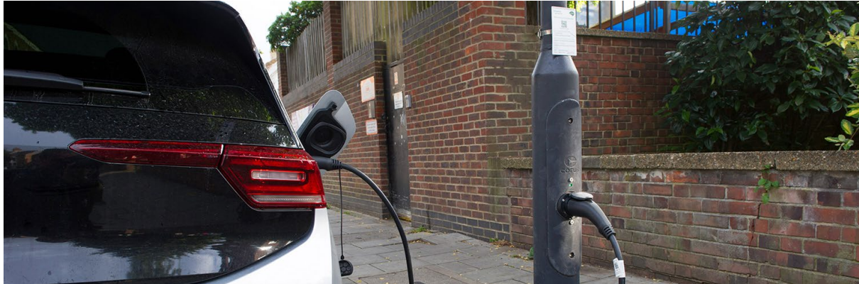
Figure 9: On-street charging devices such as converted lamp posts offer those that have an EV but no driveway the opportunity to recharge their cars within the vicinity of their home or neighbourhood
